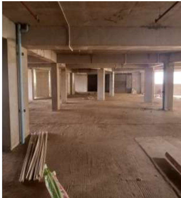
MCLP Car park
